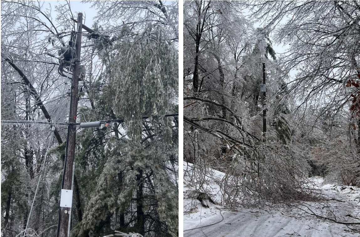
Figure 2: Damage to Electrical Infrastructure
