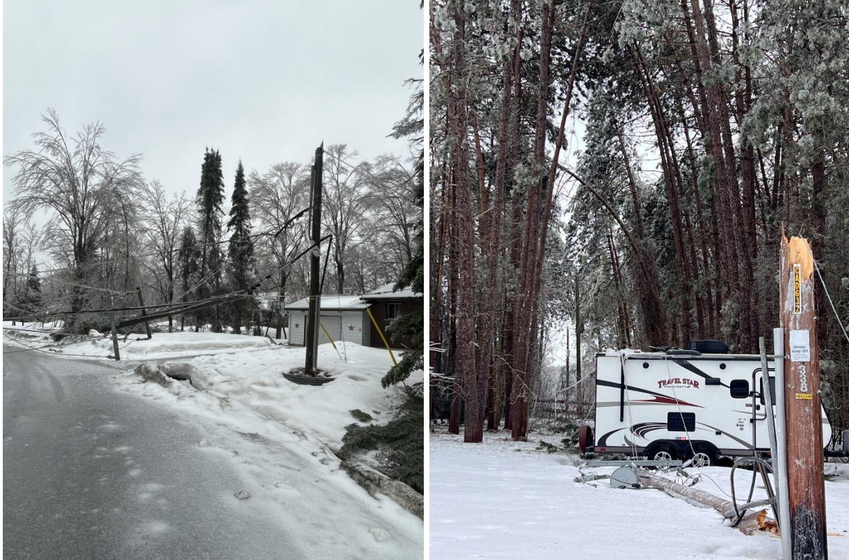
Figure 3: Examples of Broken Poles as a Result of Ice Storm Event
